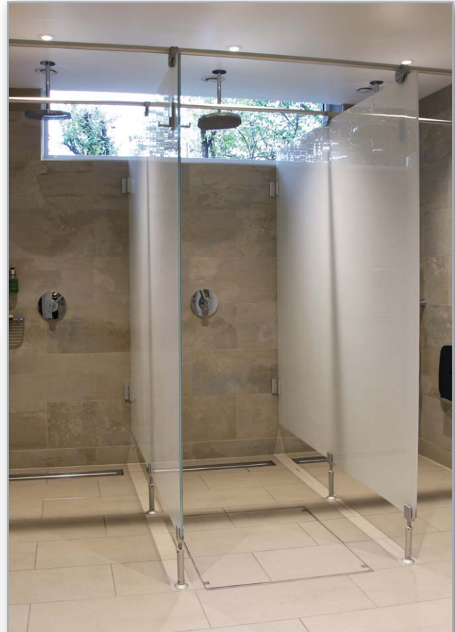
High-end bathroom, toilet, shower and cubicle installation
