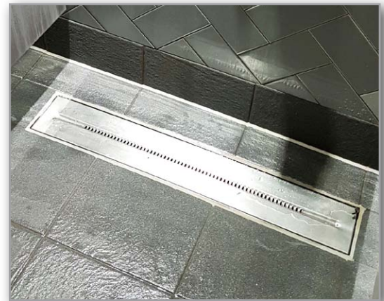
Recoup WWHRS Drain+ installed at Gymbox
