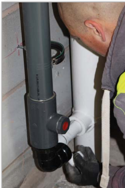
Connecting the Pipe+ HE to the soil pipe
