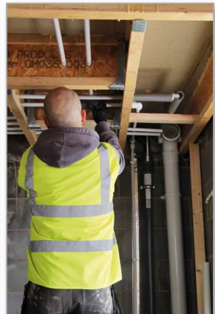
Insulation of pre-heat pipe run
